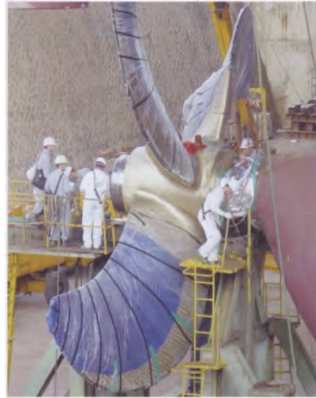
Inspectors are present during the installation of a propeller
